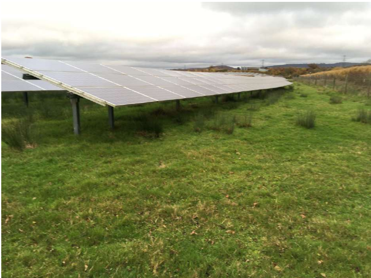
Figure 6-1 Drainage of solar panels onto grass
