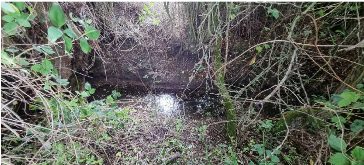
Figure 4.4 Photo of river at section 19 (taken during survey)
